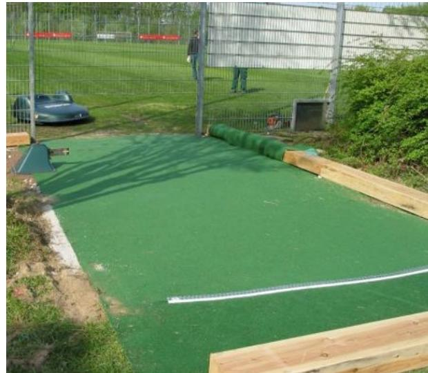
Figure 87: Charging station in narrow enclosure protected by the fence
